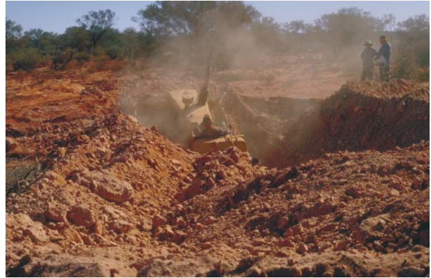
(c) Cleaning out the blast mullock from pit GCP129 with bulldozer to expose the wall sections, August 1997, view southwest. (Photo 45895)
