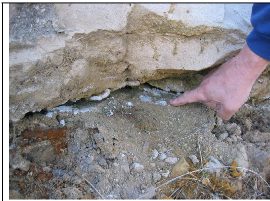
Figure 7. Close-up view of salt efflorescences in eroded cavities between the hard carbonate layer and underlying iron-rich mottled clays at site TS2, depth 140 cm.
