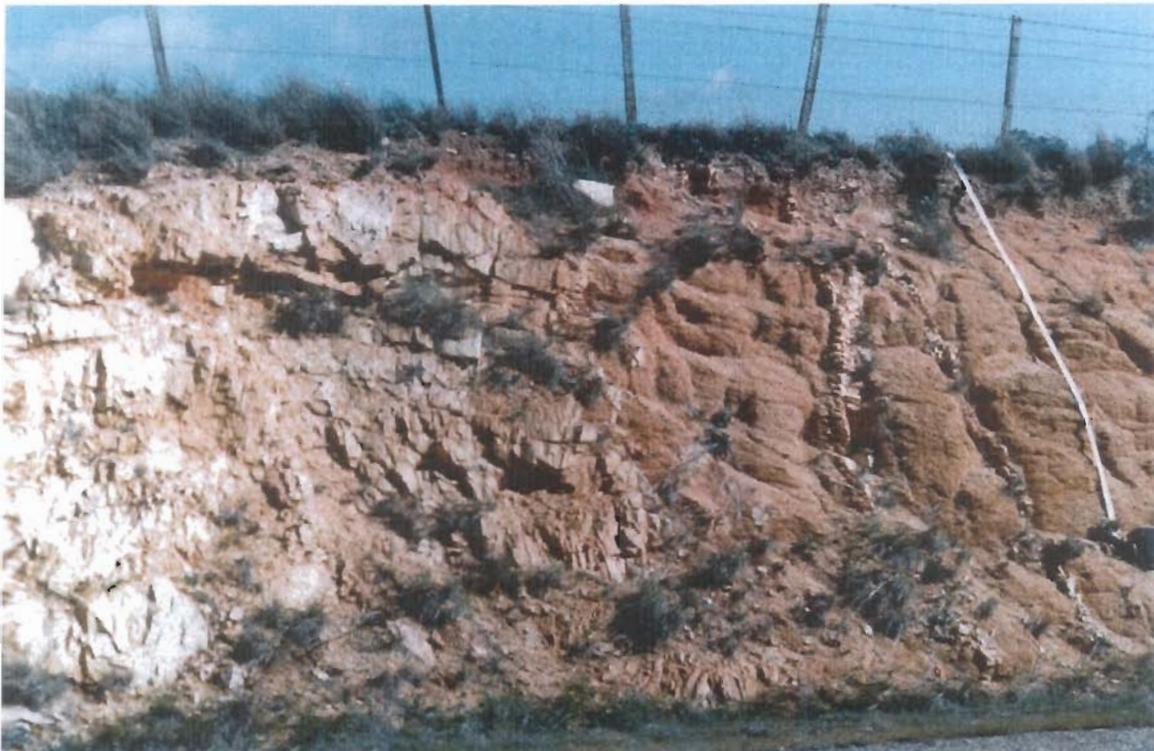
Figure 2. Sutton road cutting, showing veins through saprolite.
