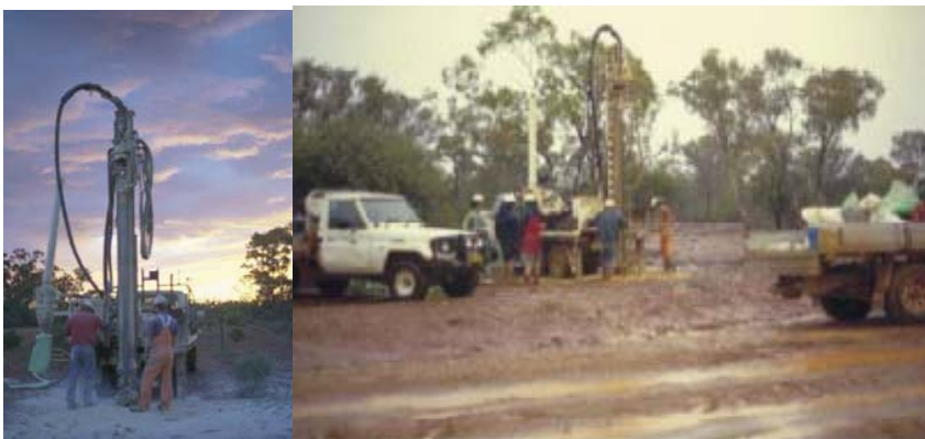
Figure 1. Air-core drilling rig in action during the Byrock Drilling Program, May-June 2003.
