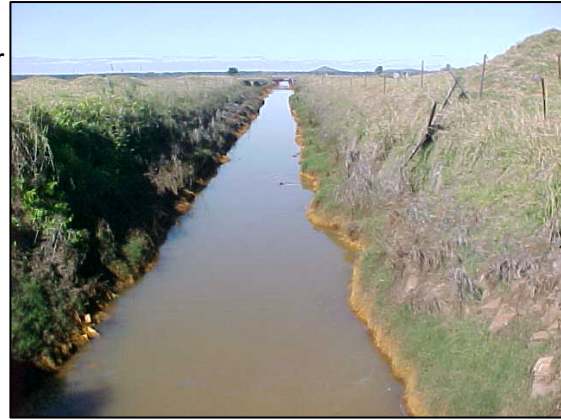
Historical deep drainage system.
