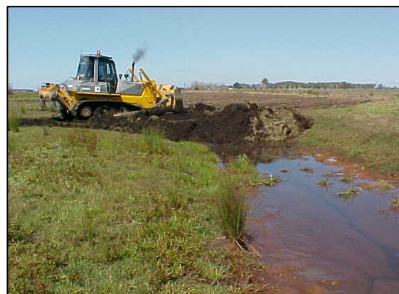
Filling in the old drain.
